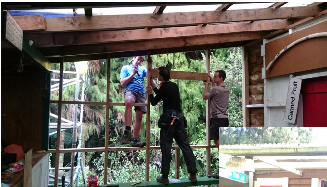
Repairing O'nuku's hut wall.
